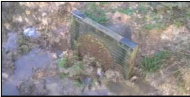
Early in the morning after a night of rain, ranger Maurice Puckett discovered that the culvert under the pest proof fence in Mangatawhiri wetland had become blocked. This caused water to spill over the bund and a whirl pool of water which undermined the pest proof fence.
