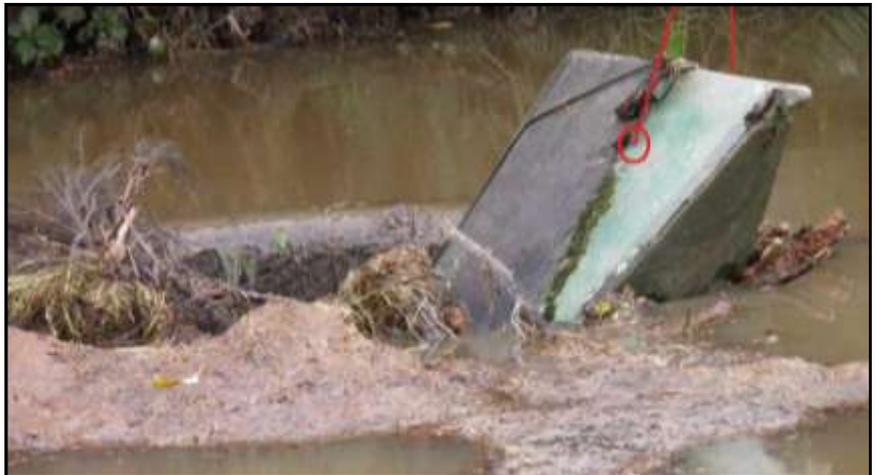
The new scruffy dome on the overflow hole on the dam blocked up with small debris and the water level rose behind the dam to flood the pump house. The pressure became so great it sucked the scruffy dome inside out down the over flow plug hole to the bottom. Eventually it was removed by a crane. (The photo on the left shows its remains.) But wait there is more! The boat used as a pateke roost got sucked down the overflow plug hole too! Lets hope the pateke were away sheltered up a bank somewhere.
