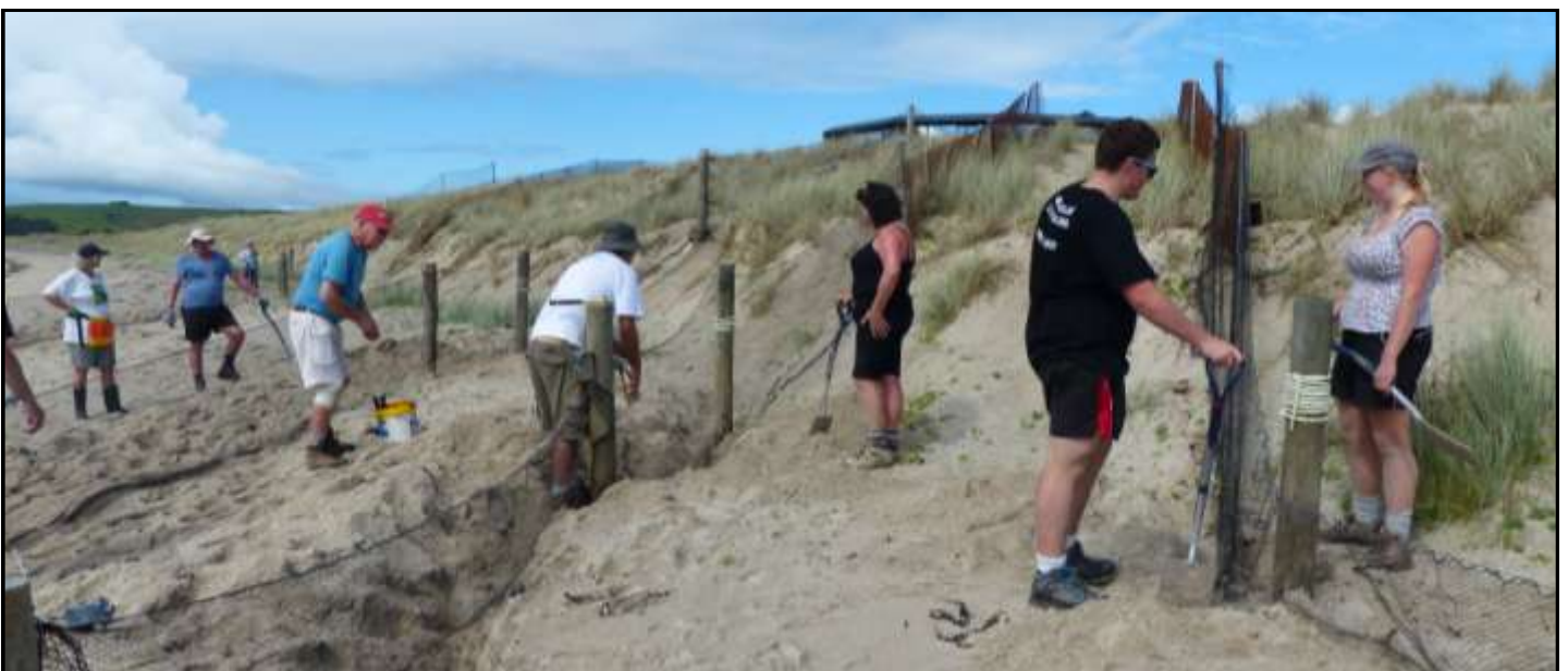
TOSSI Volunteers uncover the feathered ends of the pest proof fence, that guide critters into traps, after a storm buried them.
