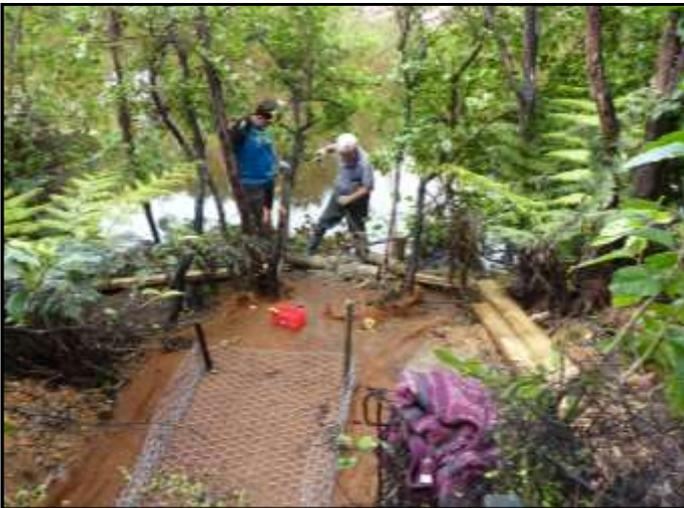
Three gabion baskets are installed to catch and filter water on the lower side of the road.
