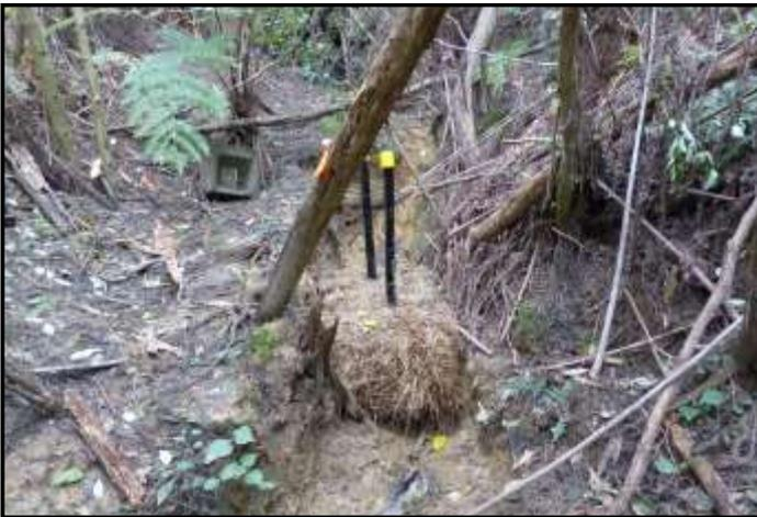
Hay bales and coconut matting were used to plug the deep gouges.
