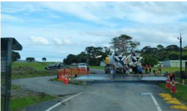
Concrete being poured for the two new gates at TOSSI. There will be a gate for in-going traffic and one for out-going.
