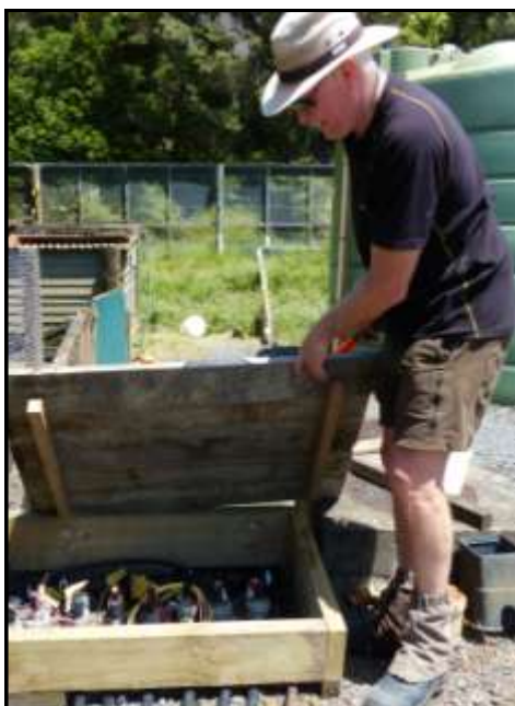
Roger Grove displays the box he built to cover the new irrigation manifold system at the nursery.
