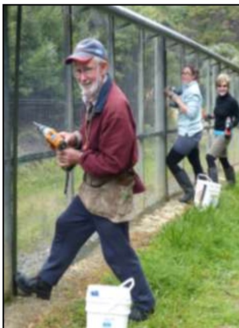
Roger Williams, with helpers Patricia and Sharon attach steel strips to the fence to strengthen the joins.
