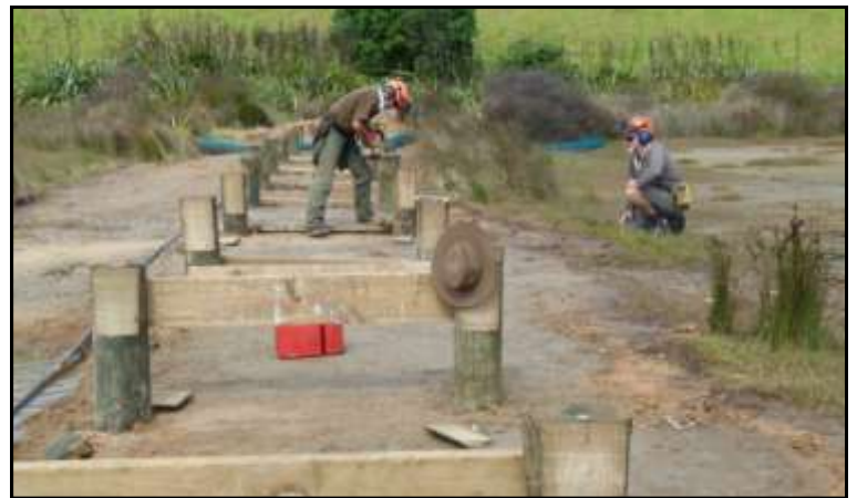
Maurice Puckett and Keith Edwards check out the levels. By removing the bund the tidal flow will be improved under the boardwalk back into the wetland.
