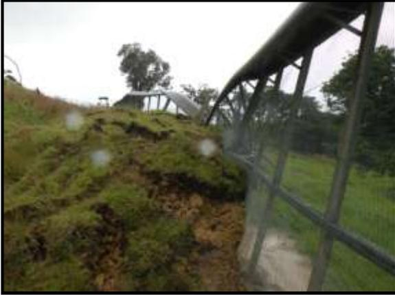
Cyclone Wilma slams the Warkworth area and sends a slip on to the pest proof fence causing a serious breach.
